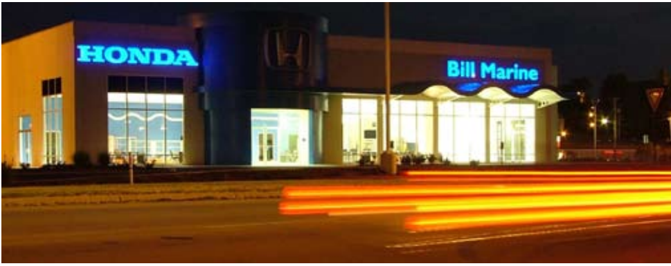
The newly constructed Bill Marine Honda dealership lights up the night in Springfield.
